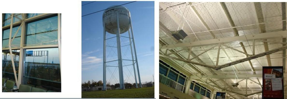
Tie Rods in Structures
